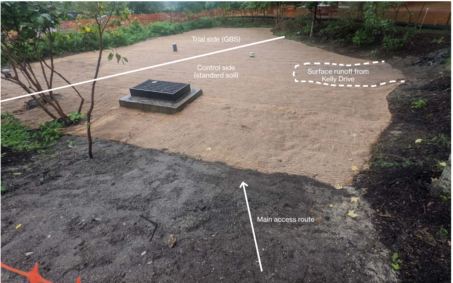
Figure 6: Access route and surface runoff from Kelly Drive entering the site.
