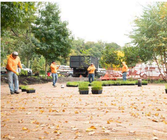
Figure 13: Installation of plant plugs.
