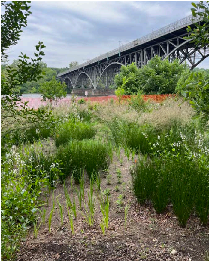
View into the bioretention basin.
