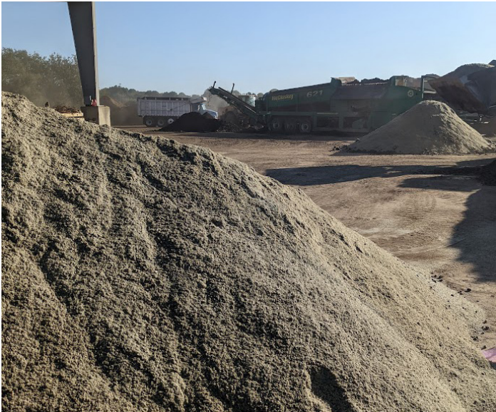
Figure 8: GBS blended at Laurel Valley Soils.
