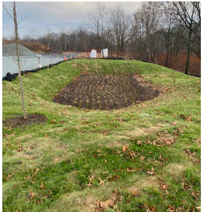
Figure 3: Rain garden with plugs and observation wells installed.
