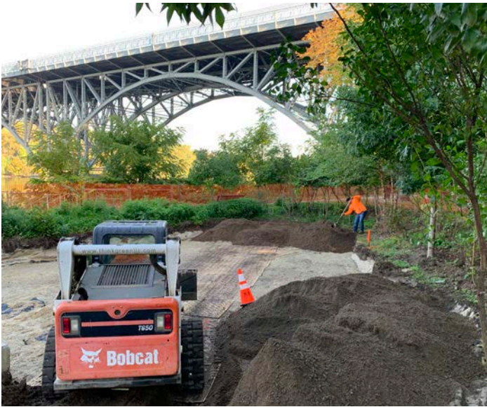
Figure 11: Excavated site with new soils for installation (credit: ThinkGreen).
