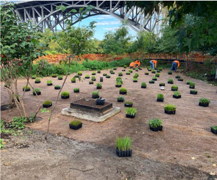
Figure 12: Laying out plugs prior to installation.
