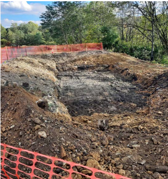
Figure 2: Rain garden under construction.
